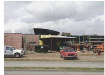
Now Under Construction: Iberia's newest rehabilitation hospital
